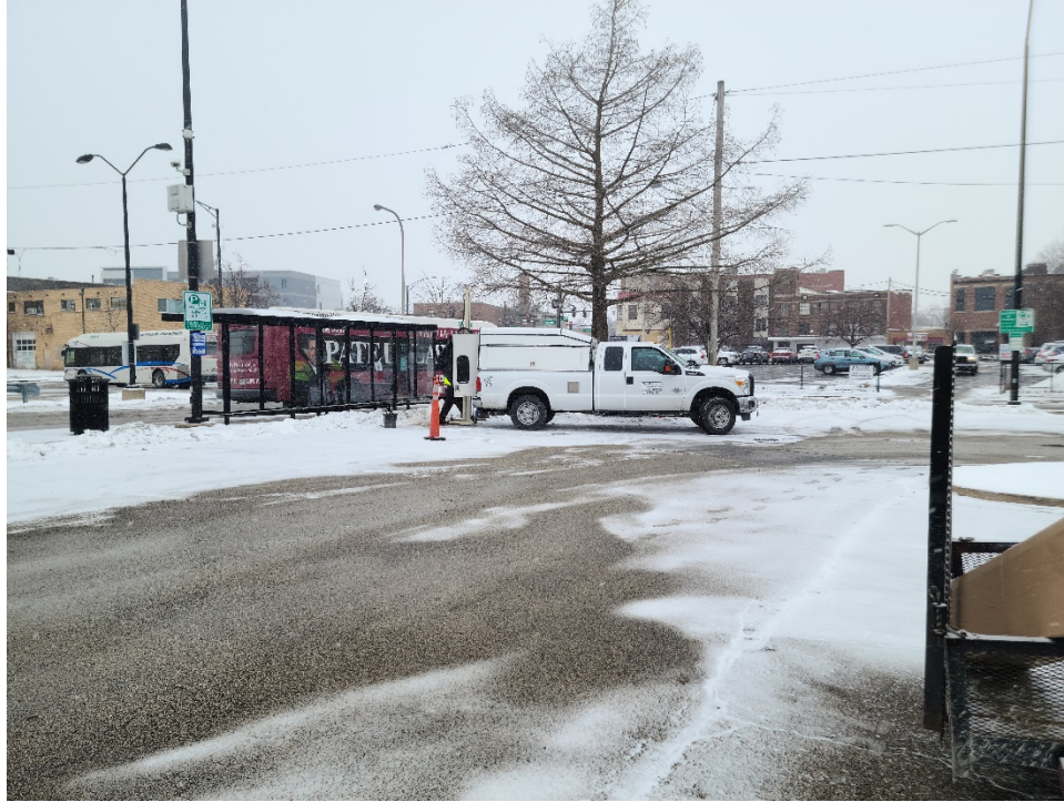
Photograph 5. Direct Push drilling at the Illinois Terminal Parking Lot
