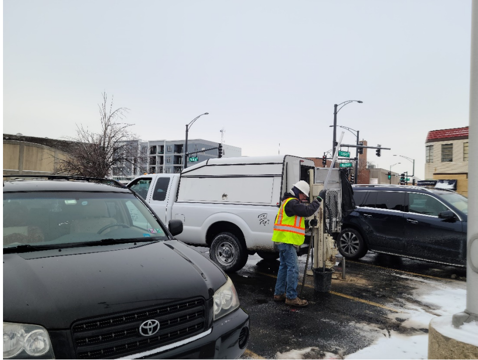
Photograph 3. Direct Push drilling at the Christie Clinic Parking Lot
