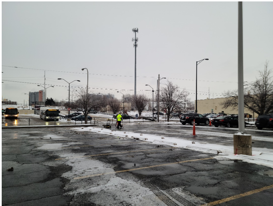
Photograph 2. Direct Push clearing soil boring locations using ground penetrating radar
