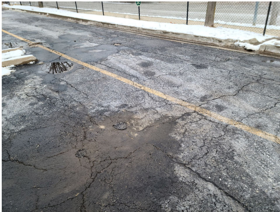
Photograph 4. Soil boring at the Christie Clinic Parking Lot backfilled
